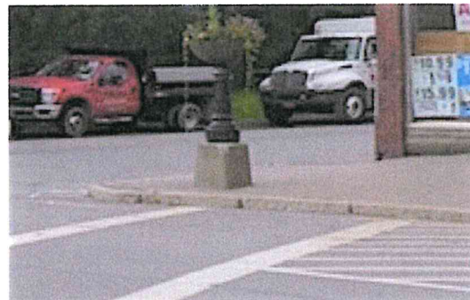
High crosswalk curbing is not wheelchair friendly (Stewart Avenue, Roscoe)
