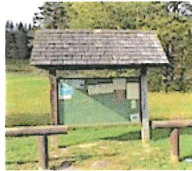
Underutilized State roadside kiosk (Route 81)
