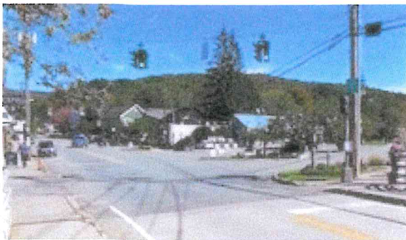
Unmarked intersection crosswalks (Main Street, Livingston Manor)
